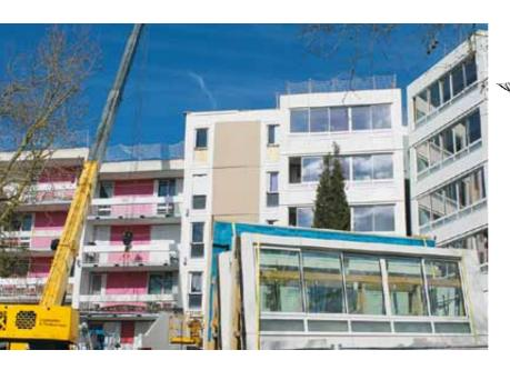
Thanks to a Savings Funds loan, 494 flats in the Beaulieu district of Poitiers are being retrofitted. The aim is two-fold: to obtain the BBC Rénovation retrofit label and install solar panels that will supply power for the hot water and heating networks. The retrofit project is taking place between 2013 and 2015 in an occupied setting.
